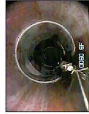
CCTV Video Testing
